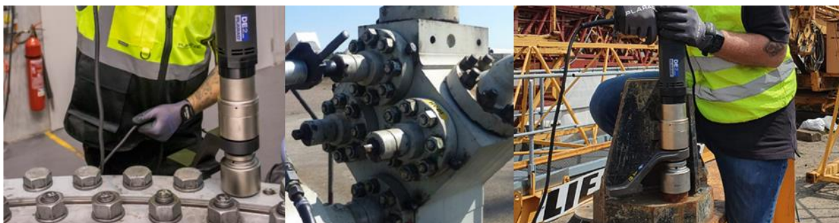
Bolting solution with the electric torque wrench DE1 on gate valves
